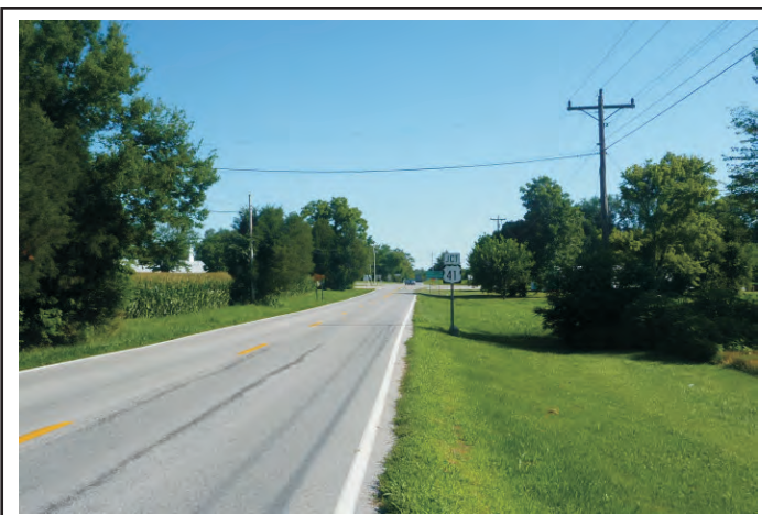
Photo 23: Representative photograph of existing roadway configuration, KY 181 at US 41, facing south.
