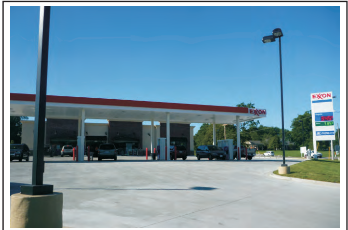
Photo 16: Hazardous materials concern site Property ID 3, Beach Oil (dba Exxon #25) at 11945 Guthrie Highway (KY 181) with active UST record, facing north.
