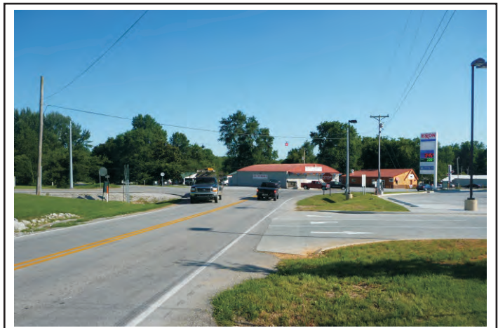
Photo 18: Potential location of hazardous materials concern site Property ID 5, South Todd Turning Lanes at Guthrie Road (KY 181 at US 79) with an inactive CWA record, facing south.
